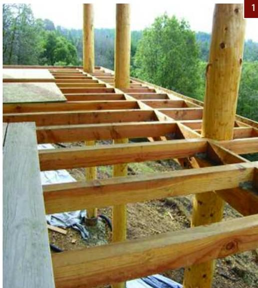
1 Frame deck with 4" joists 23 7/8" on center
