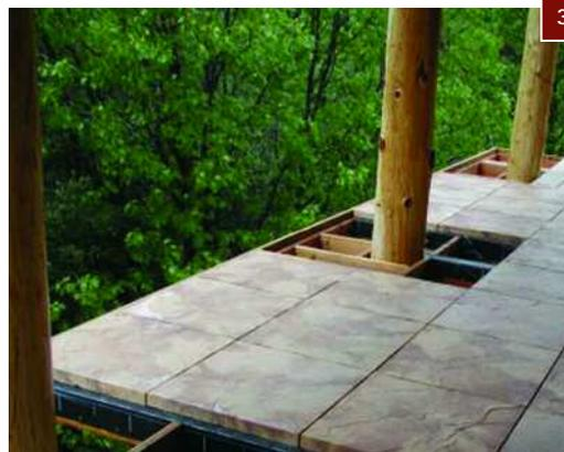
3 Simply lay Dekstones on joists
